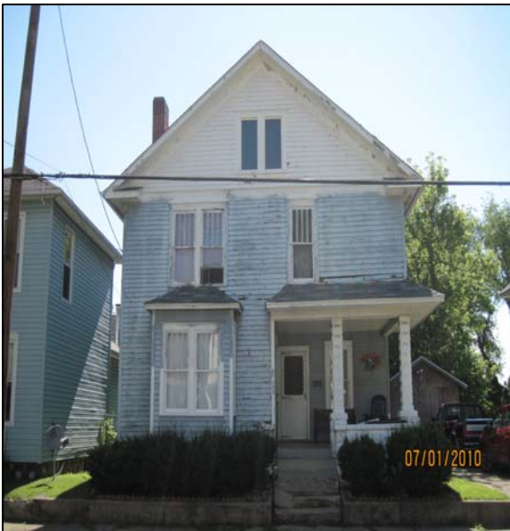
Left: Neighborhood eyesore before lead remediation & rehab.
