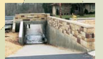
Tunnel at Granville Street
