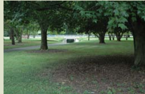
Tunnel at Licking View Drive
