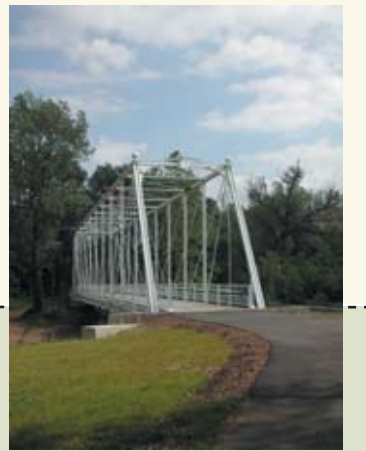
Gallman Bridge at Cherry Valley Road
